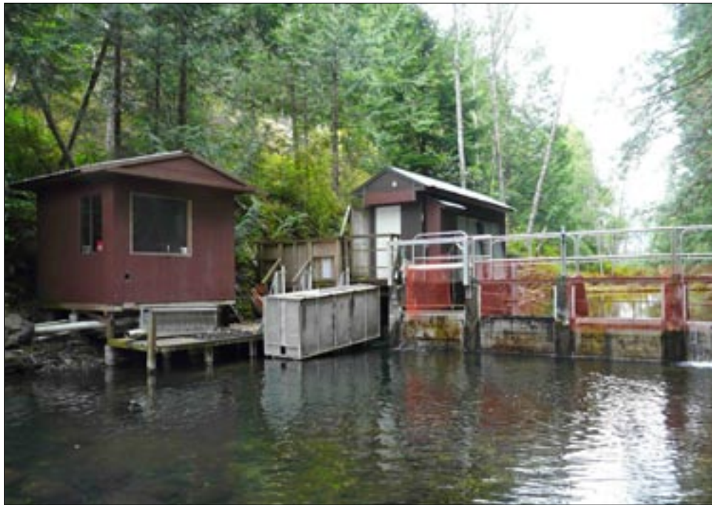
Salmon smolt can be diverted to a holding tank and counted at this small dam and fishway, located on the stream connecting Sakinaw Lake to the sea.
