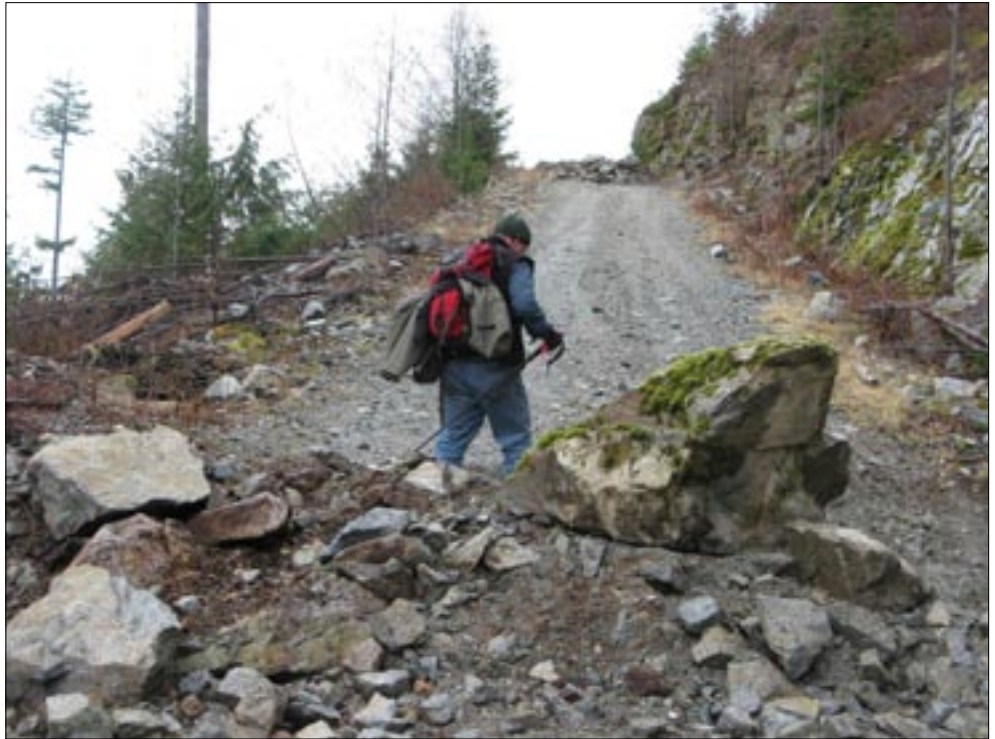
An example of Plutonic's road deactivation on Mount Troubridge.
